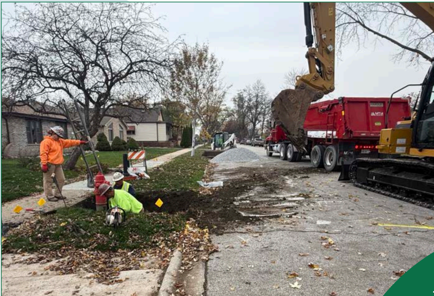
Priority community hydrant replacement during construction
